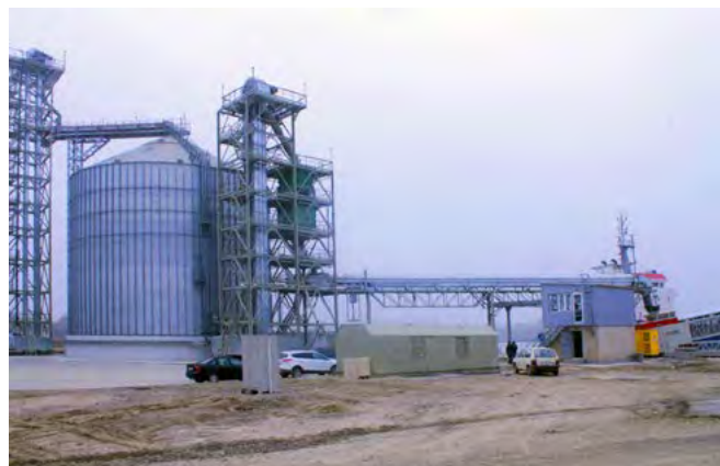
Trans Cargo Terminal (Trans-Oil Group)
